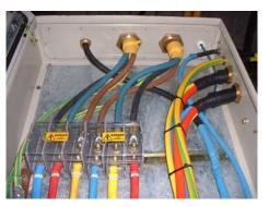
Figure A-2 - Junction box connections
