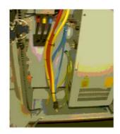
Figure A-3 - Cable tails common at Variable frequency converter
